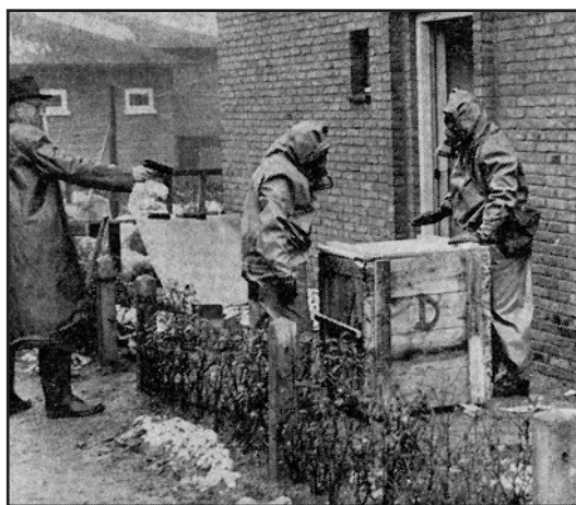
Figure 13. The concrete drums with radioactive debris are packed in wooden cases. Note the man pointing with a Geiger counter.
